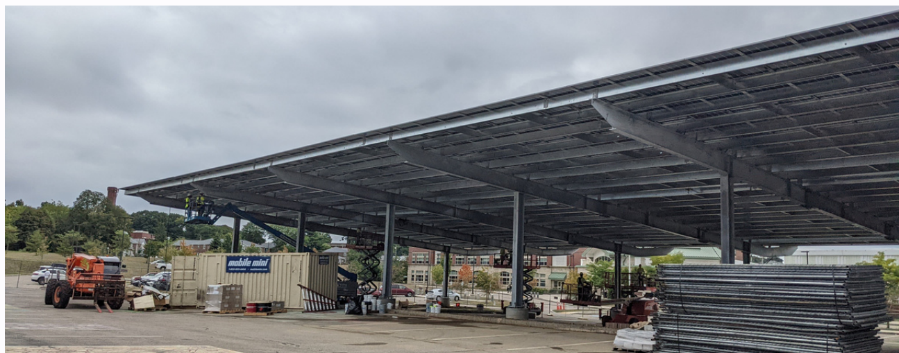
Solar canopies under construction at Beverly High School, Aug. 23, 2022
