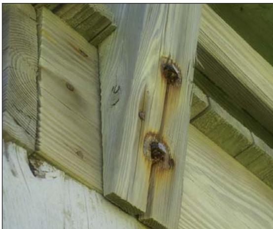
**Deck disaster?** This is not an atypical condition of the materials and connections for decks built near the ocean. Heat, ultraviolet light, elevated moisture levels, and salt spray exact a stiff toll on wood decks in relatively short periods. A condition like this should raise safety concerns for both the deck builder and the general contractor.
