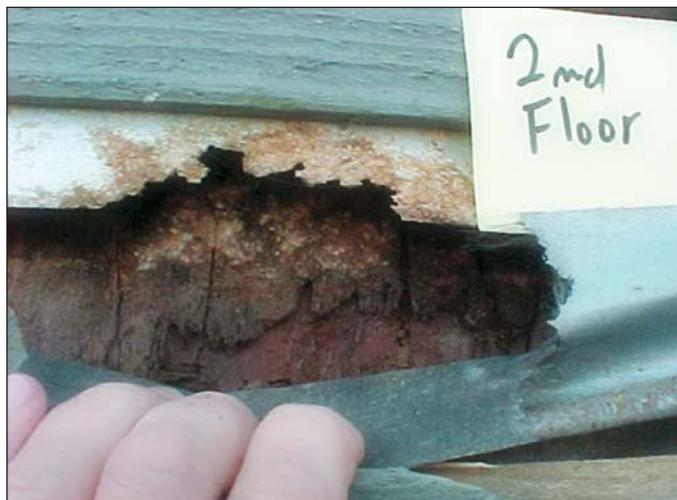
**Premature decline.** On a beachfront home in Virginia, no Z-type flashing was installed over the ledger-to-house connection, which led to extensive decay.
