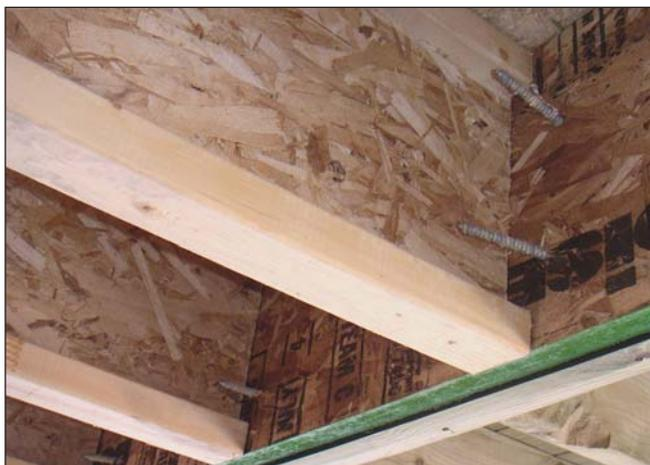
**Wrong!** Deck joists (framed with PT framing lumber) have been hung from a ledger that is lagged into the rim board of a cantilevered I-joint system. Even if the lag screws were to be positioned to penetrate the I-joint flanges, the connection would be dangerously weak. It is likely to collapse under very low loads, possibly the dead load of just the deck structure itself. DCA6 strictly prohibits the connection of a deck to a cantilevered overhang.
